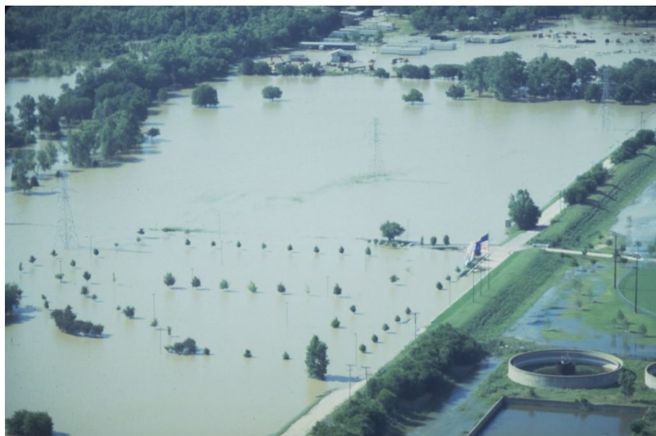
Figure 1.22: Flooding, Trinity River Levees
